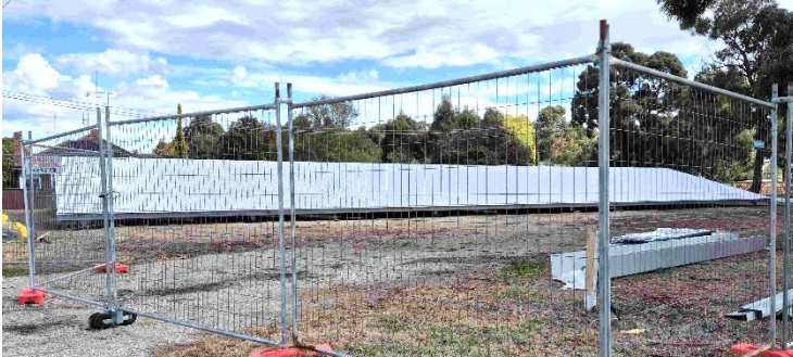
The roof complete and waiting for the lift
