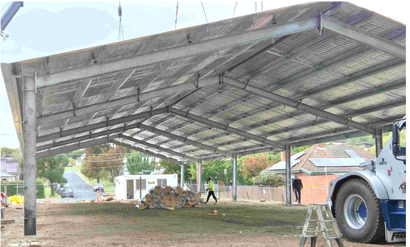
It only took a few minutes to lift and it's actually beginning to look like a building
