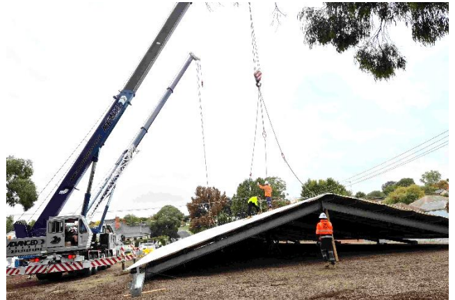
Cranes in position – ready for lift off!
